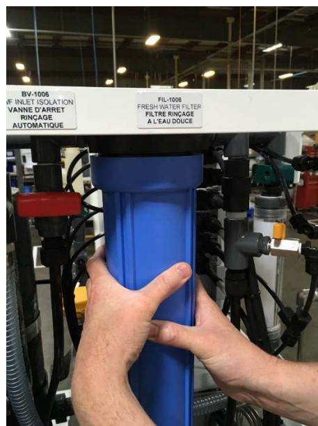
Figure 7.5 - Installation of Fresh Water Filter
