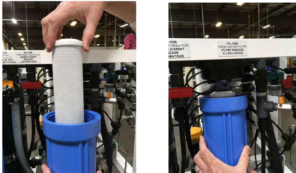
Figure 7.6 – Installation of Fresh Water Filter (Cont'd)
